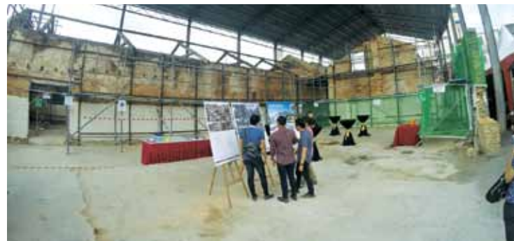
The current state of the interior of the godowns as seen here. Once restored to MSC compliance status, they would have all the state-of-the-art facilities of a modern office.
