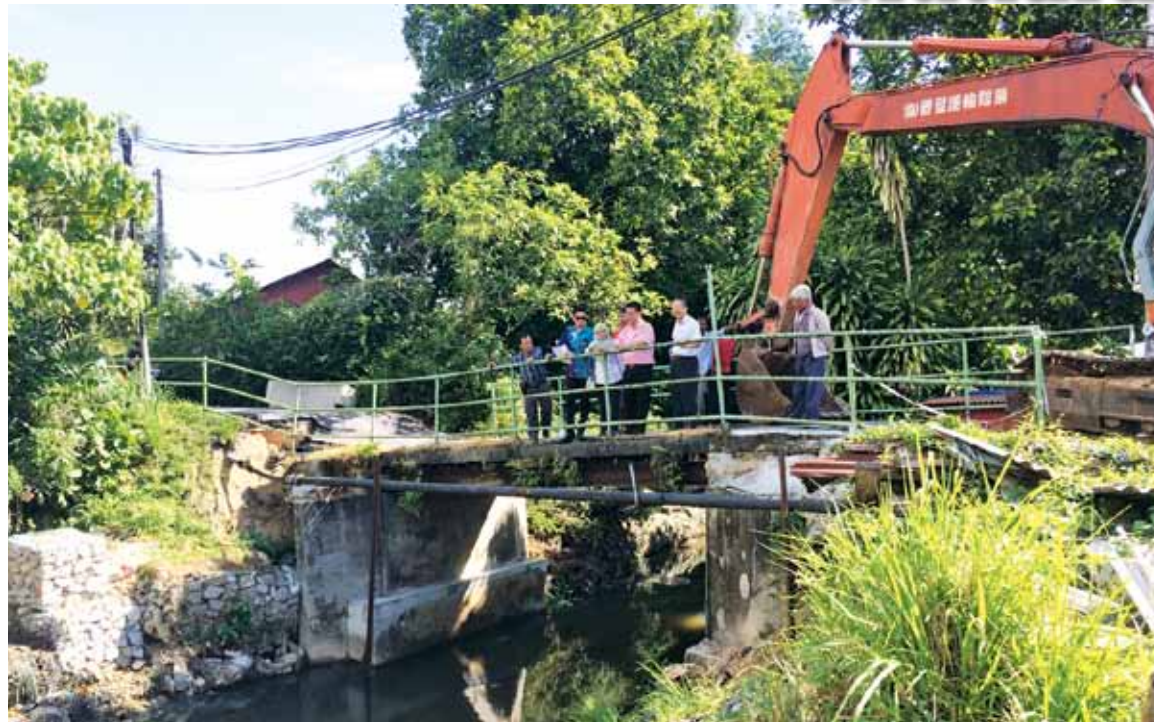
Wong (in pink), Nortilawati (third from left) and other officers looking at the condition of the damaged bridge connecting Solok Zoo 1 and Tingkat Lembah Ria 1.
