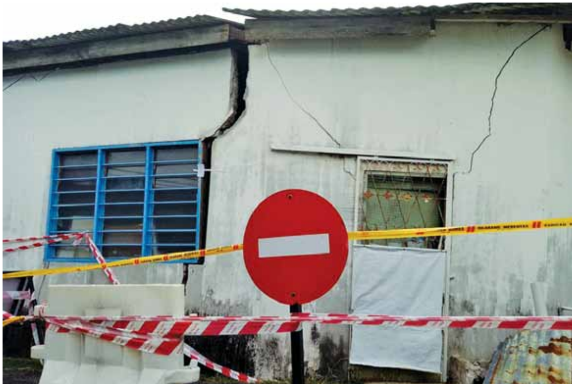
One of the affected houses in Hong Seng Estate.
