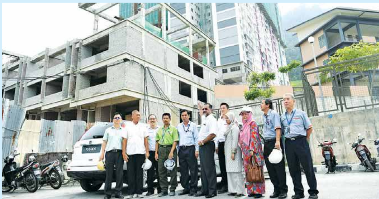
Jagdeep (sixth from left) pointing to a Dua Residensi apartment block under construction as other guests present during the site inspection look on.
