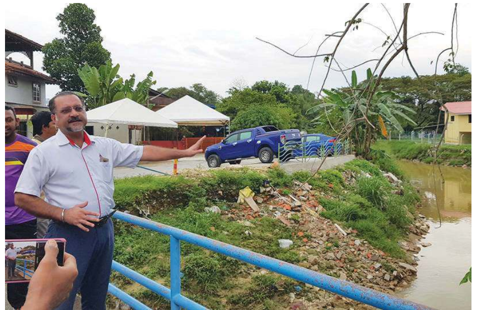
Jagdeep pointing to the ‘worrying condition’ of river bank.
