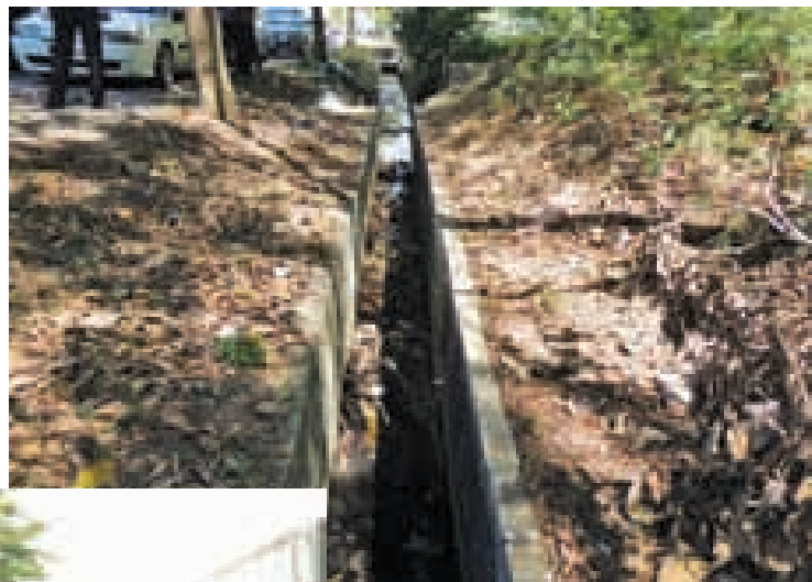
Part of the scupper drains that would be re-constructed.
