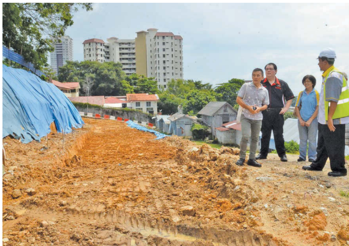
Teh (first from left) inspecting the site where the connecting road is being built. Standing behind him is Lee.
