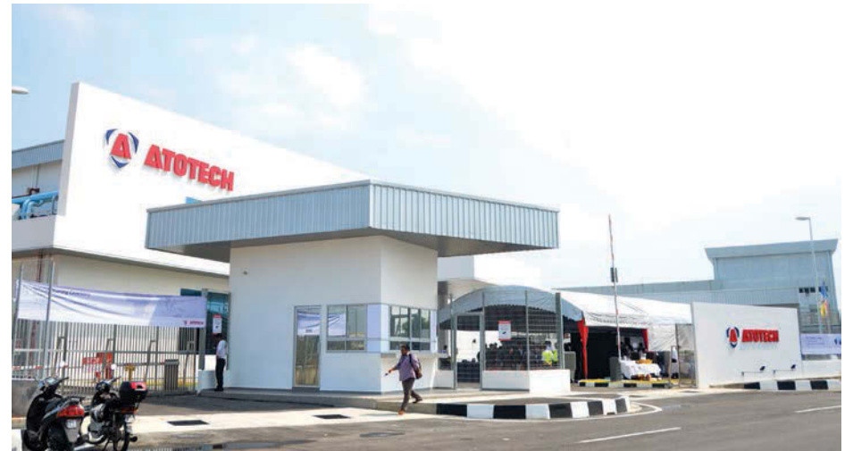
The new Atotech chemical plant at Batu Kawan.
