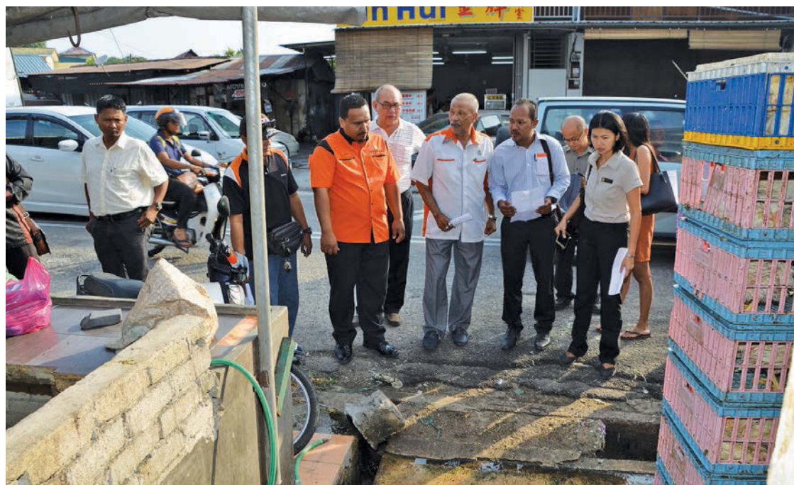
Gan (right) with Mohd Harani (fourth from left) checking out the condition of the drains at the Bayan Lepas market.
