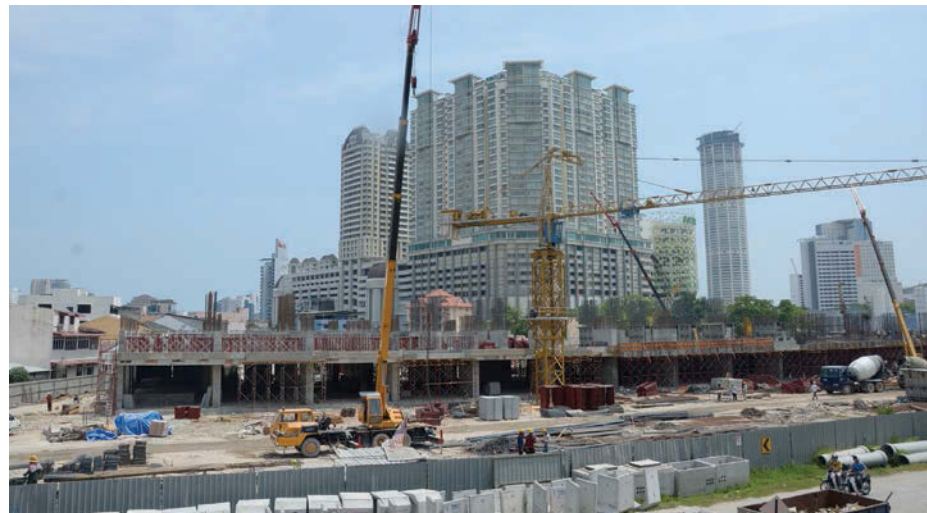
SP Chelliah housing project under construction.
