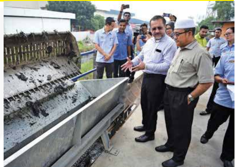
Jagdeep and Rozali discussing how the pump houses work in Perai Industrial Area.
