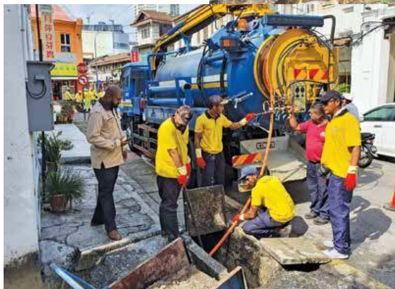
MBPP workers using a hydro jet to flush away grease and dirt from a clogged drain in Jalan Pintal Tali in George Town.
