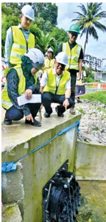
Sarimah (squatting, left), Wong (squatting, right) and others inspecting the drainage system at the site.
