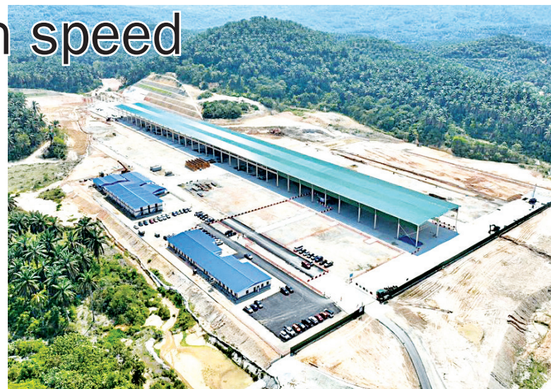
A drone shot of the 38-acre SBG casting yard in Kulim.
